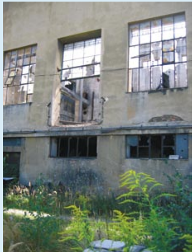
Fig 3.1., 3.2 Sidings of steelwork plant and ancillary buildings in Krakow. Photos: archive IURS, author Y. G. Garb.
