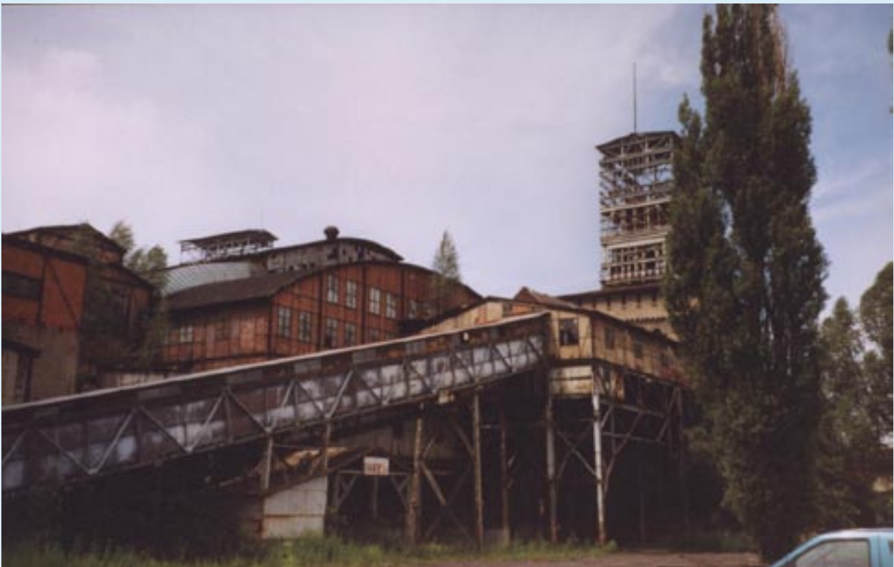
Fig. 6.2 Processing plant and monumental tower of the Julia shaft in Wałbrzych (Poland) converted into museum of technology
