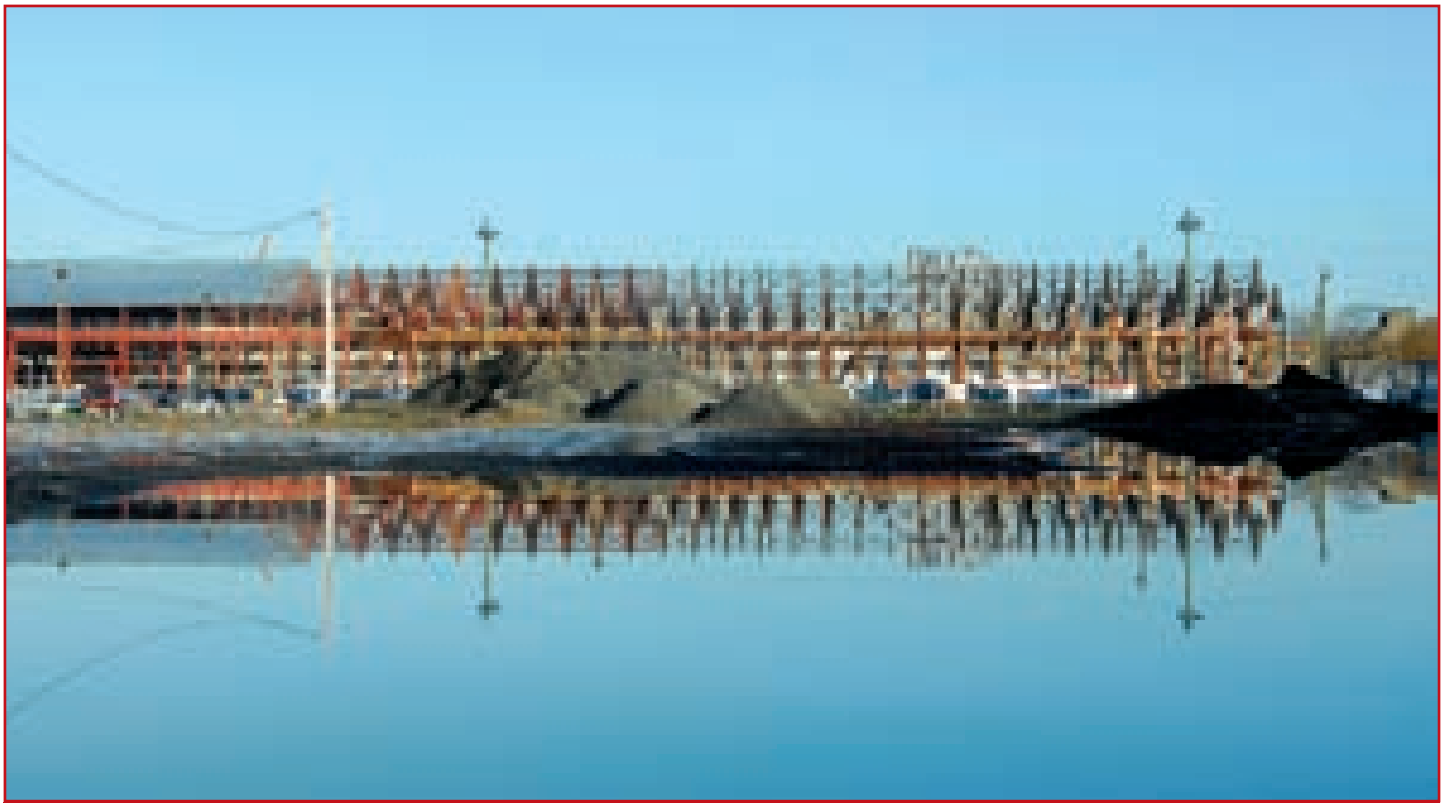
Future "Nef Dubigeon" under construction
