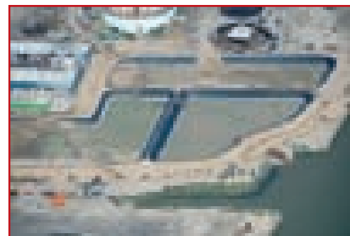
Settlement ponds: land remediation - Rochester Riverside
