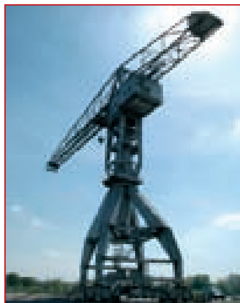
The Grey Titan Crane on the former Nantes Shipyards site - Île de Nantes
