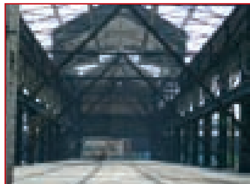
Former Stork–Dijkers foundry undergoing renovation – Hengelo
